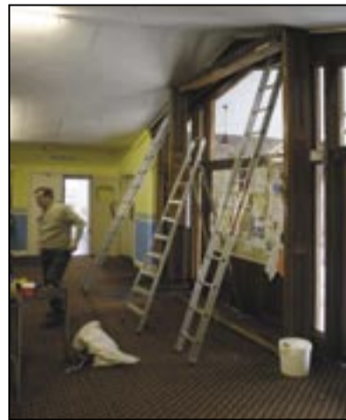
The first banner case under construction
